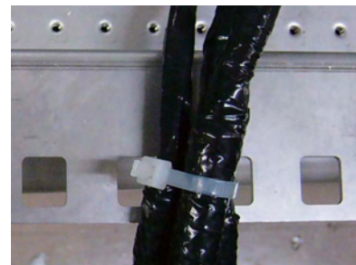
Fix cables to post with cable tie
